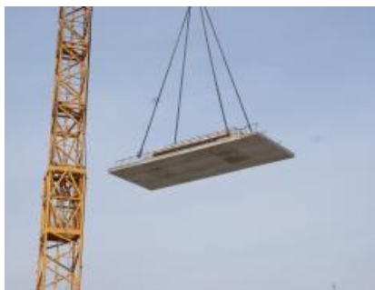
Figure 23 A floor slab
